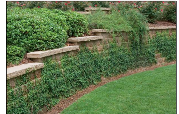
Example of a Reinforced Segmental Gravity Walls (Manufactured Modular Concrete Units)
