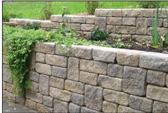
Example of Reinforced Segmental Gravity Walls (Manufactured Modular Concrete Units)
