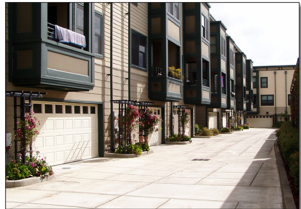
AN URBAN ALLEY BEHIND A MIXED-USE TOWN CENTER DEVELOPMENT.
