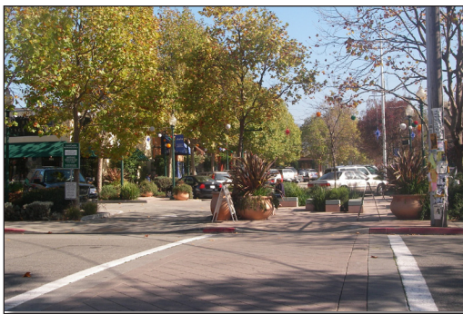
Special Pavement Markings Delineate This Pedestrian Crosswalk
